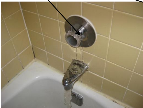
Shower faucet is leaking. Sink pipes are leaking.
