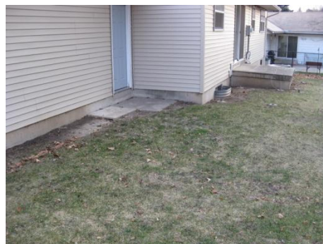
Areas on the west and south yards have negative sloping. Recommend adding fill to bring grade back to a positive slope.
