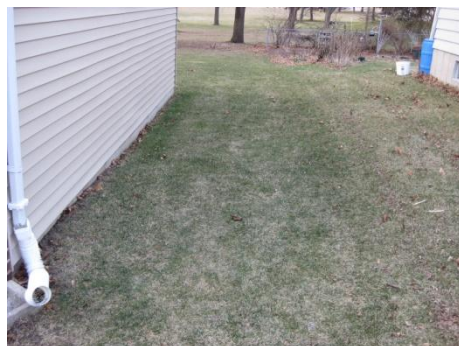
Areas on the west and south yards have negative sloping. Recommend adding fill to bring grade back to a positive slope.
