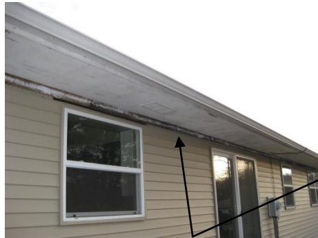
Areas of siding missing on south and west sides.
