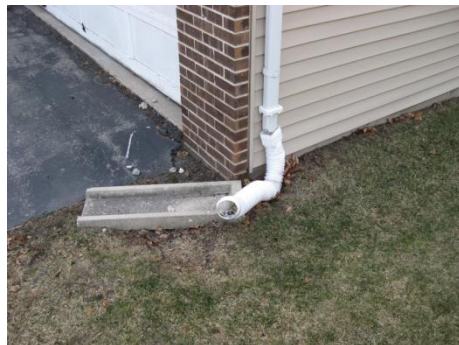
Recommend extending downspout extensions at least 6 feet away from house.
