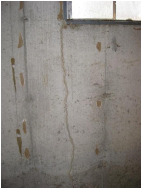
Basement south foundation wall crack. Recommend monitoring each of the foundation cracks for continued movement and further evaluation/repair if necessary.
